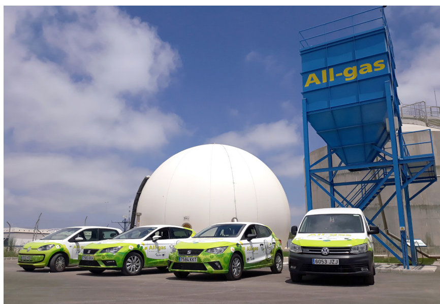
All-gas is a worldwide pioneering project that is revolutionizing the paradigm of wastewater treatment by obtaining clean energy in a sustainable way from effluents.
