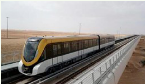
The first train circulation tests of the main line in manual mode
